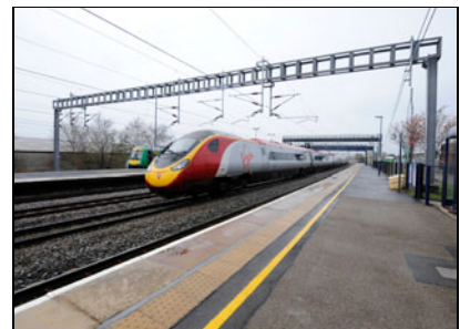
Bethell Rail Platform extension at Tamworth
