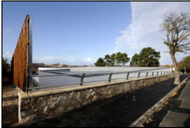
Bethell Construction Aldi Stores, Colwyn Bay
